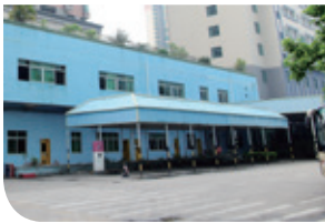
Location: Administration Building
