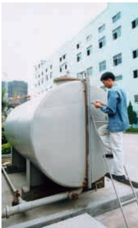
Regular checking on fuel storage for in-house power generator 定期測量廠內發電機之燃油儲備
